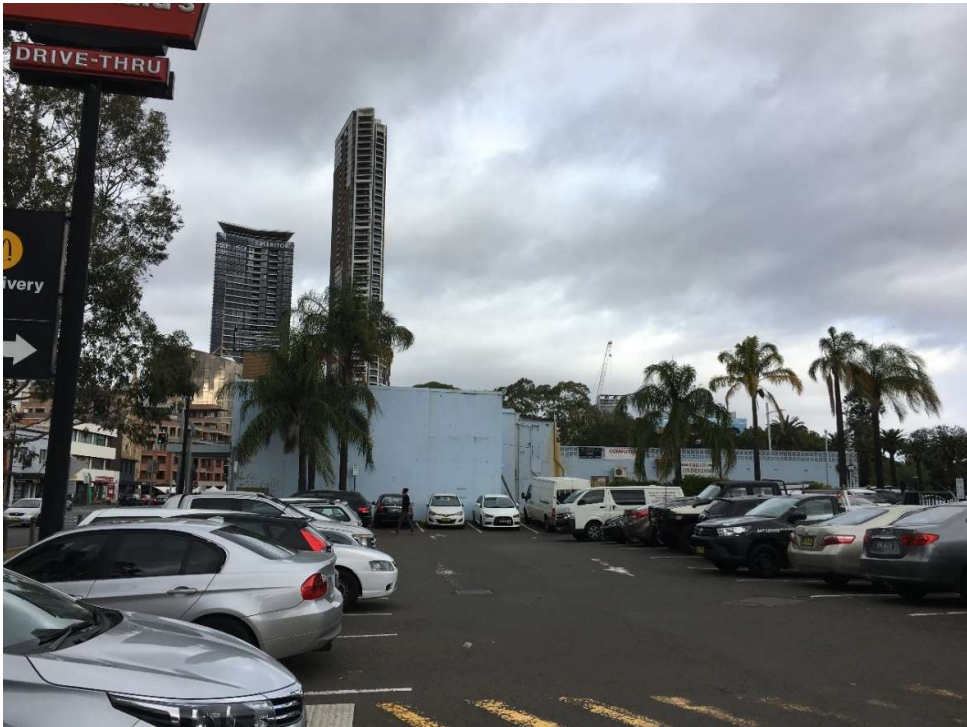
Figure 17: View looking south across the McDonald's carpark to the vacant commercial buildings at 355 Church Street.
