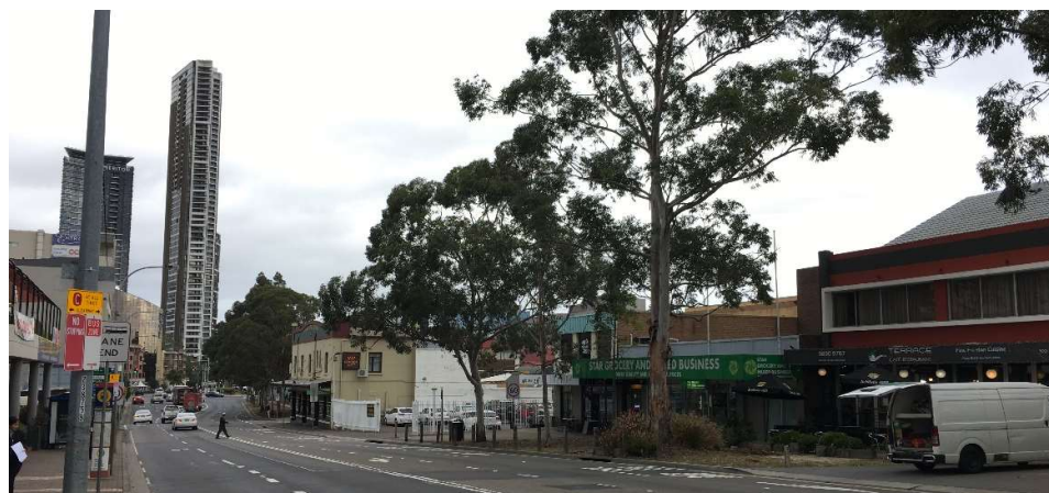
Figure 30: View 6 - looking south along Church Street from the south east corner of Grose Street shows the inconsistent building set backs on the western side of the street. Future development on the subject site will be seen in the background of this view, in the context of the high rise development existing and under construction in the evolving city centre.
