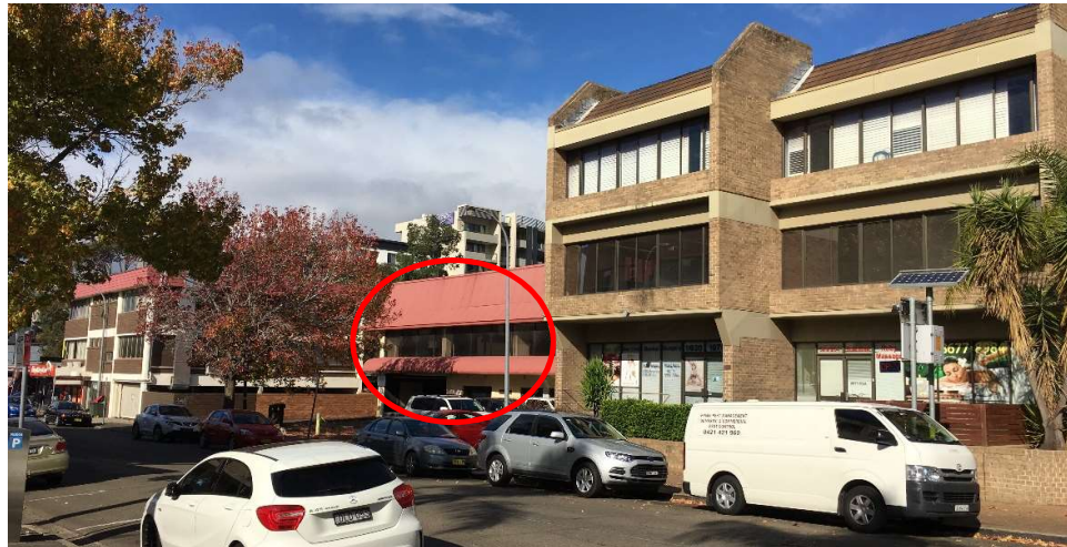
Figure 48: View from the footpath outside 14 Ross Street includes the subject site (marked with a circle) and the existing development at 385 Church Street, to its left, and that at 5-7 Ross Street, to its right.
