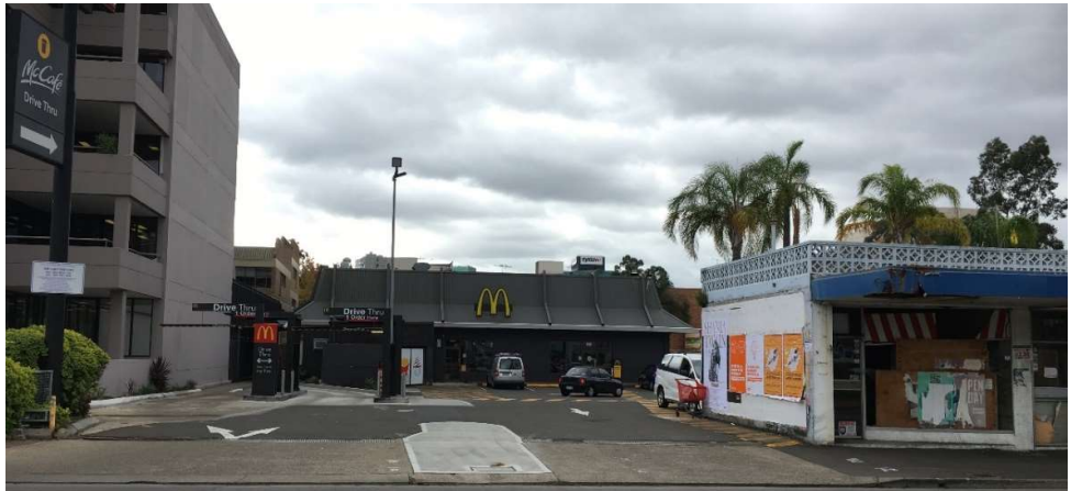
Figure 16: The Victoria Road vehicle entry and exit to the site.
